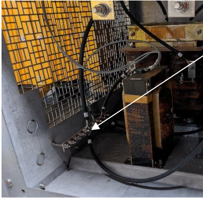
Ground Bus in a free-standing NEMA 3R enclosure
